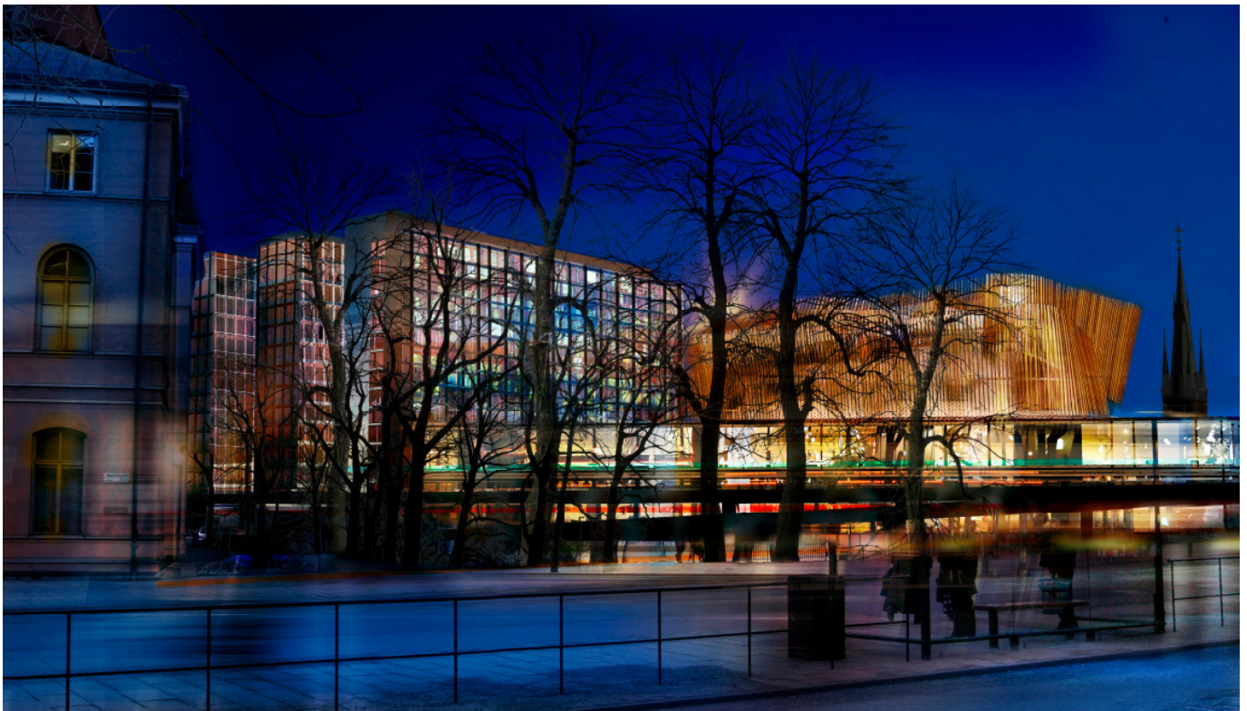
Figure 3: Stockholm Waterfront. A steel construction made from 2000 tons of construction steel and 65 tons of stainless steel. It has advanced energy solutions resulting in energy usage for heating and cooling of half the limit for a green building.[19]
